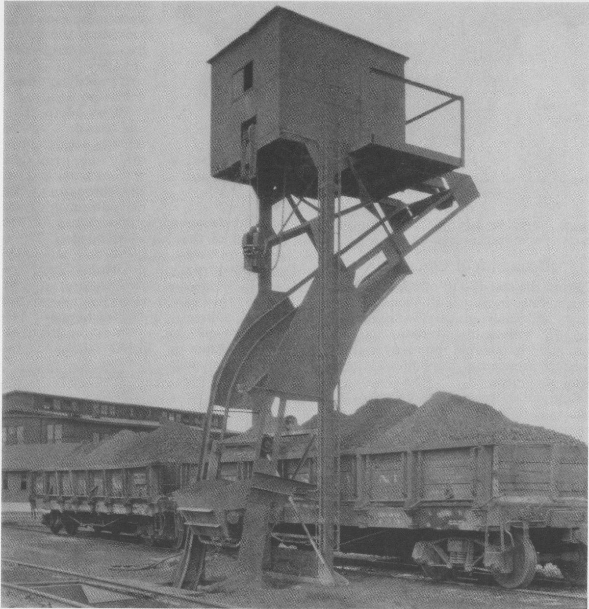
Cinder conveyor at Pratt, Kan., one of ten units installed for the Chicago, Rock Island & Pacific Railway. This conveyor is electrically operated and serves two tracks. It is controlled from the push-button station located on the side of the tower
