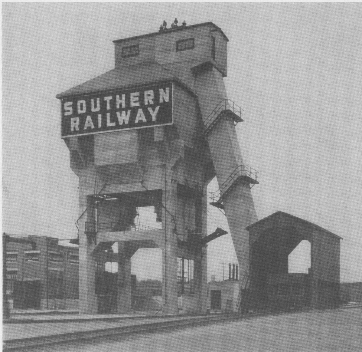
A capacity of 800 tons is provided in this coaling station built for the Southern Railway at Atlanta, Ga. Coal is served to the tenders on three tracks from the platforms. Two scales, with 15-ton scale pockets and type-registering beams, give printed records of all coal issued
