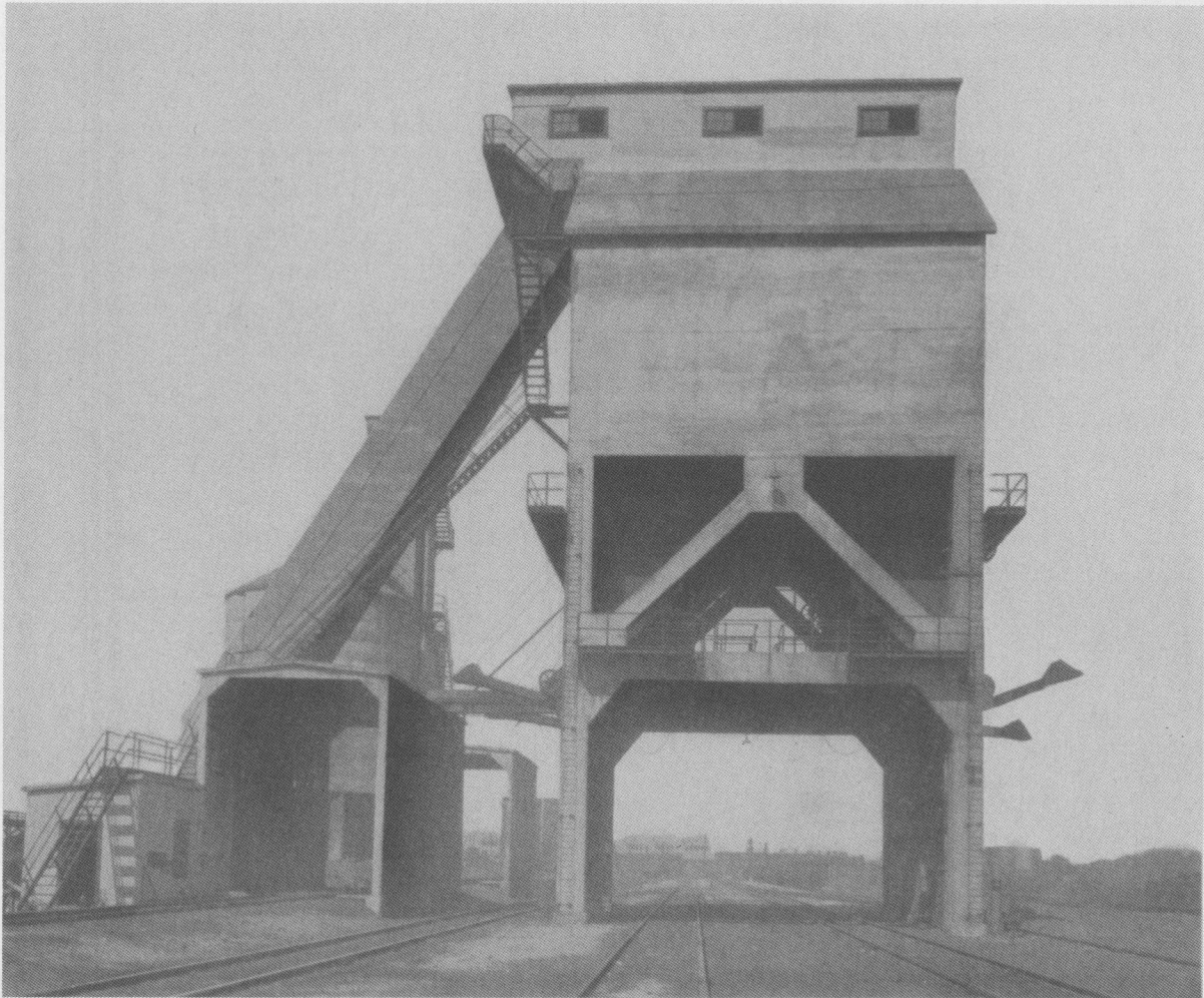
Coaling station and sand plant at Shopton, Iowa, one of the 54 Fairbanks-Morse stations on the lines of the Atchison, Topeka & Santa Fe Railway Co. The coaling station has a capacity of 1,000 tons, serves four tracks, and is equipped with four 15-ton scales for weighing all coal issued. The sand plant is exceptional in that it provides storage for a six months' supply
