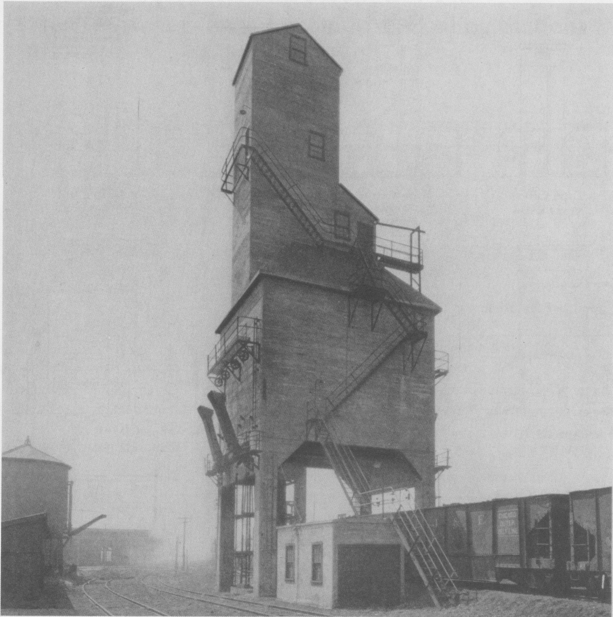
A 500-ton automatic skip-hoist coaling station installed for the Elgin, Joliet & Eastern Railway at Waukegan, Ill. This station serves two tracks, is operated with electric drive, and has a crusher located just above the storage pockets
