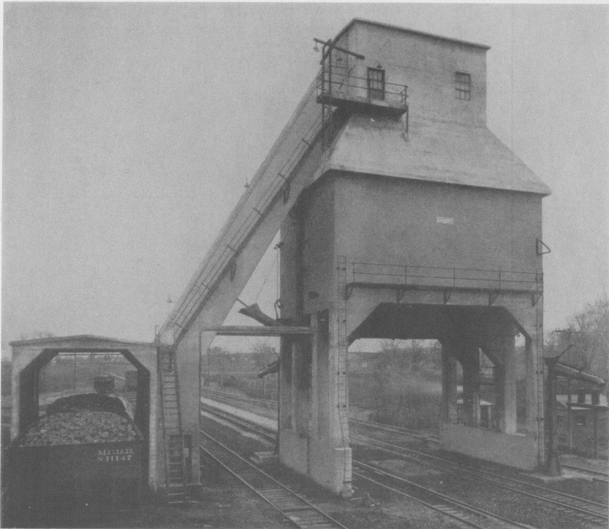
The 500-ton locomotive coaling station, on the Michigan Central Railroad at Augusta, Mich., is a typical modern station. Situated halfway between Detroit and Chicago, it enables locomotives on the main line going in either direction to take on coal and water at one stop and in less than one minute
