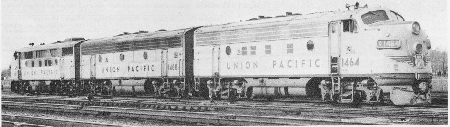
The F7 played a relatively small role in UP's dieselization (only 18 A's and 34 B's), lost among 179 F3's and 344 GP9's. Even the 88 FA/FB1's outnumbered the F7's, unlike on most roads. It should be pointed out, though, that UP's 28 1550-series Phase IV F3's have F7-style full length stainless steel grills and can be easily confused with F7's. Two of those 18 F7A's, 1464 and 1465, were rebuilt from wrecked F3A's (1504, 1553) in 3-4/52. Above, 1464/1488C/1417 wait at N. Platte, NE, about 1954, just before the influx of GP9's.
